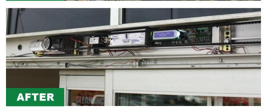
Example of replacing all the drive components and wear items with the DC One Sliding Door Retrofit.
